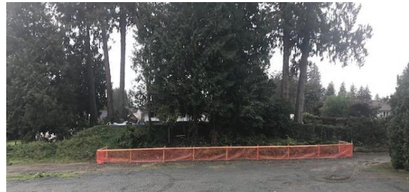
Example of protective tree fencing
